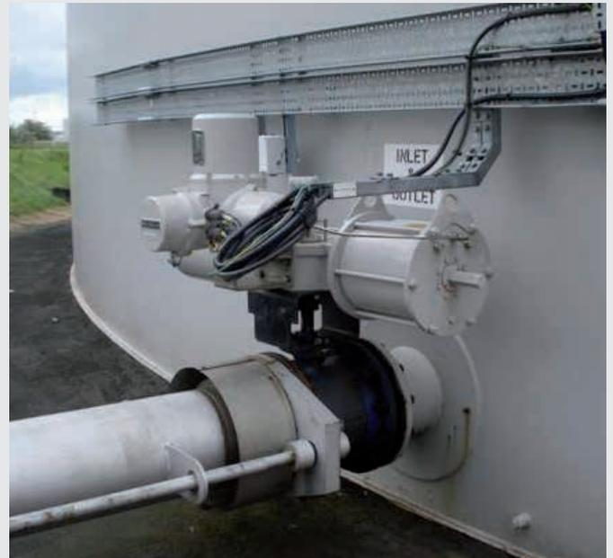
**Figure 2:** Triple excentric butterfly valve ZWICK TRI-CON used as ESD-Valve on a storage tank in Scotland
