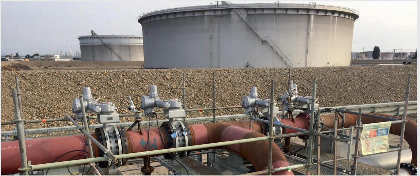
**Figure 3:** Tankstorage pipeline system with TRI-CON butterfly valves
