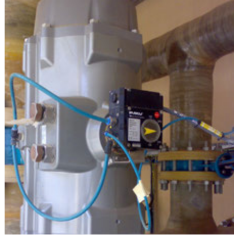
EP5 on large quarter turn actuator
