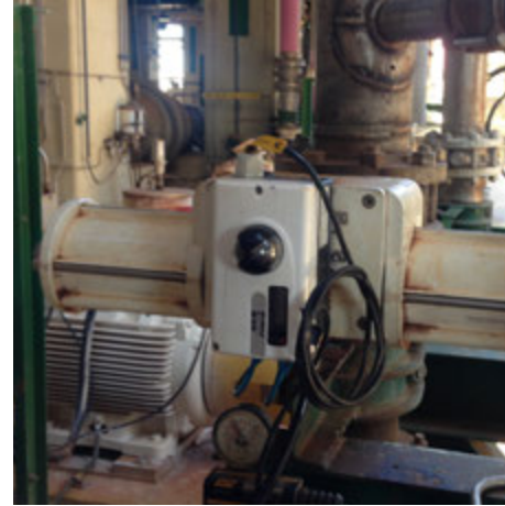
D30 Digital positioner on NAF control valve
